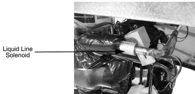
Figure 52. Liquid Line Solenoid (1 per barrel)
