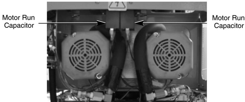
Figure 45. View of Motor Run Capacitors
