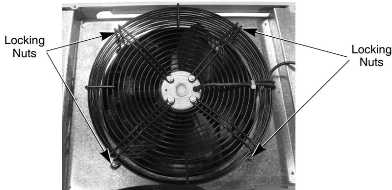
Figure 50. Condenser Fan Mounting Nuts
