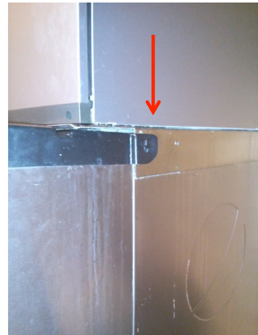
Effect: Adapter not sealed results in external mineral deposits
