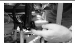
25. Check all connections on the Expansion Tank for leaks.
