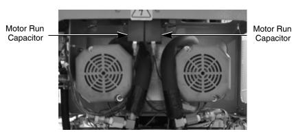
Figure 45. View of Motor Run Capacitors
