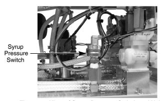
Figure 53. View of Syrup Pressure Switch and Valve
