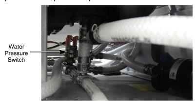
Figure 54. View of Water Pressure Switch
