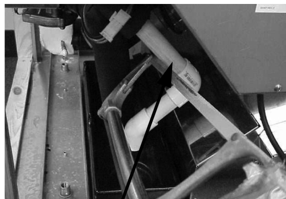
Cut PVC Drain
