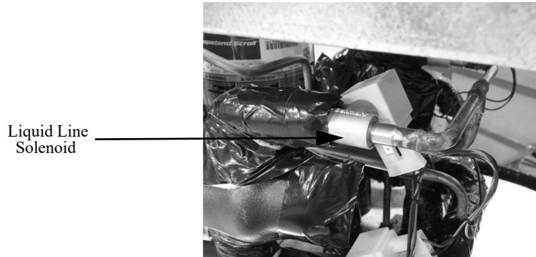
Figure 78. Liquid Line Solenoid (1 per barrel)
