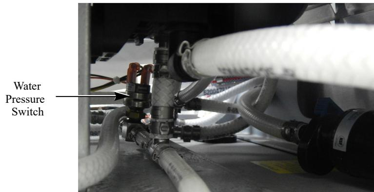
Figure 80. View of Water Pressure Switch
