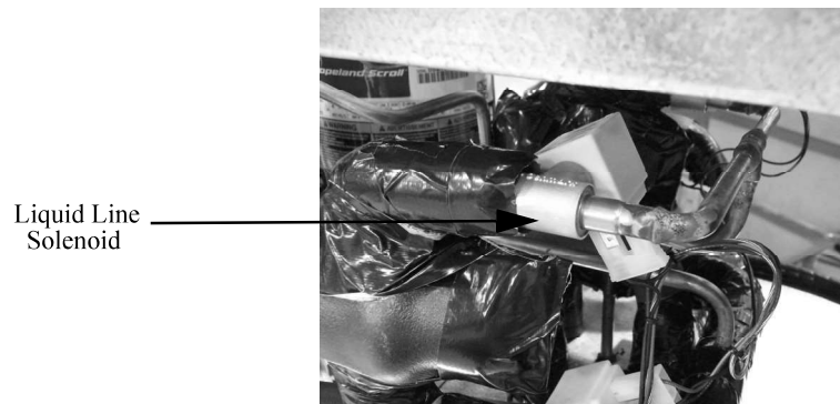
Figure 55. Liquid Line Solenoid (1 per barrel)
